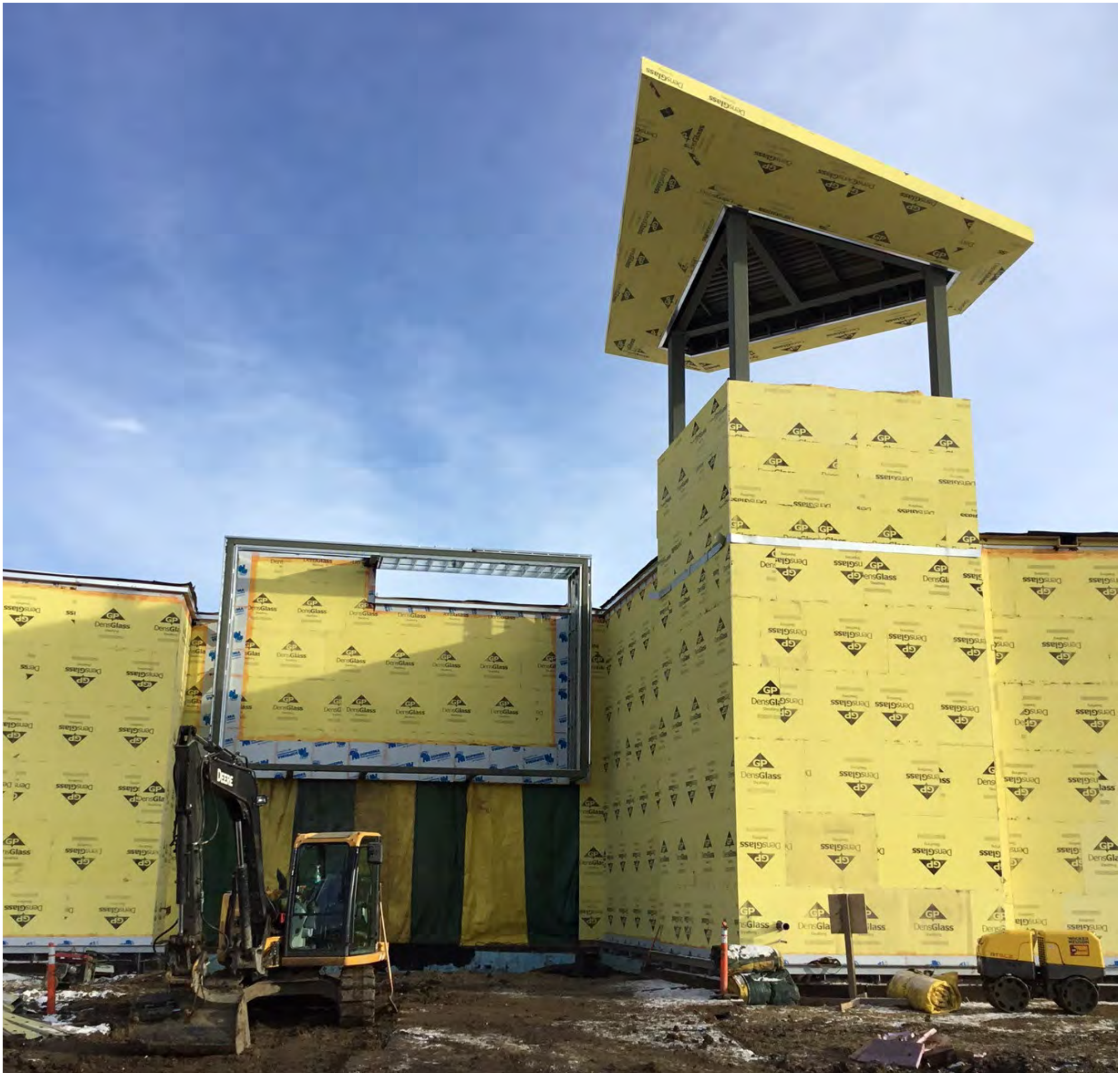
EDMONTON CONSTRUCTION - ENTRY
